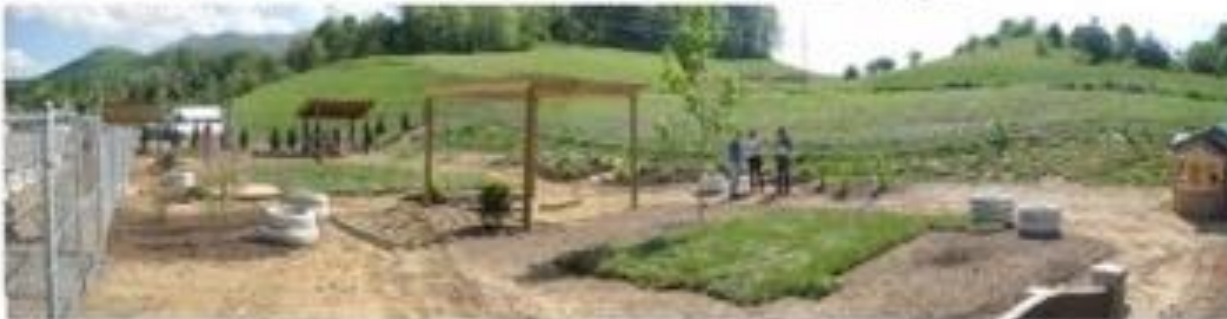
AFTER: Genesis Academy in Burnsville, NC - 2010, play area improvements in progress
